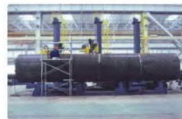
■ Circumferential seam welding
